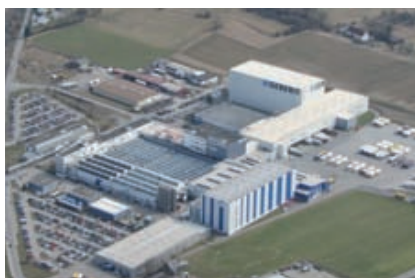
The new central distribution centre in Pfullendorf (Southern Germany).
